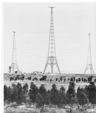
The Naval Radio Transmitting Facility, Chula Vista, California, as it appeared upon completion in 1917. "This is a high-powered radio station and contains three 600-foot steel towers, with necessary power house, office building, shop, water tank, main barns, four quarters for operators and quarters for the officer in charge." - Rear Admiral Roger Weller, first Commandant of Naval Operating Base, San Diego, 1920.
